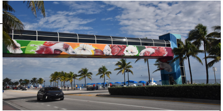
STC tinted The Westin Fort Lauderdale Beach Resort's beachfront pedestrian bridge and elevator with 15% net tint transmittance.
